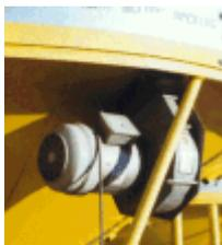
A typical aeration cooling fan mounted on an elevated grain silo.
